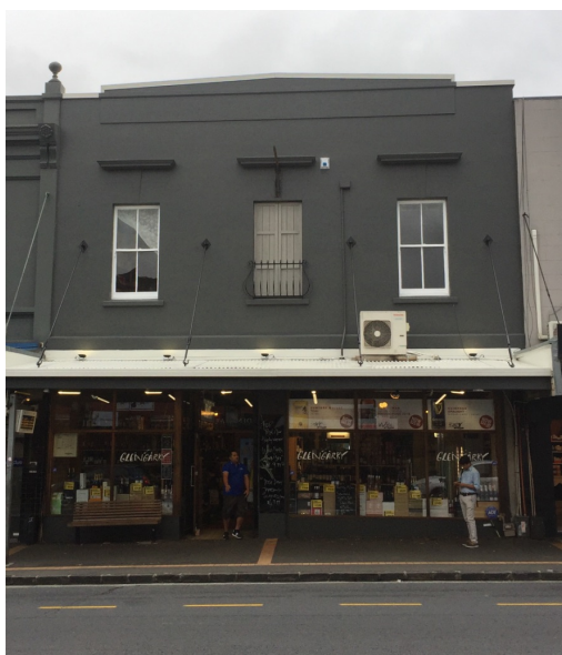
Figure 3: Mt Eden URM Building
